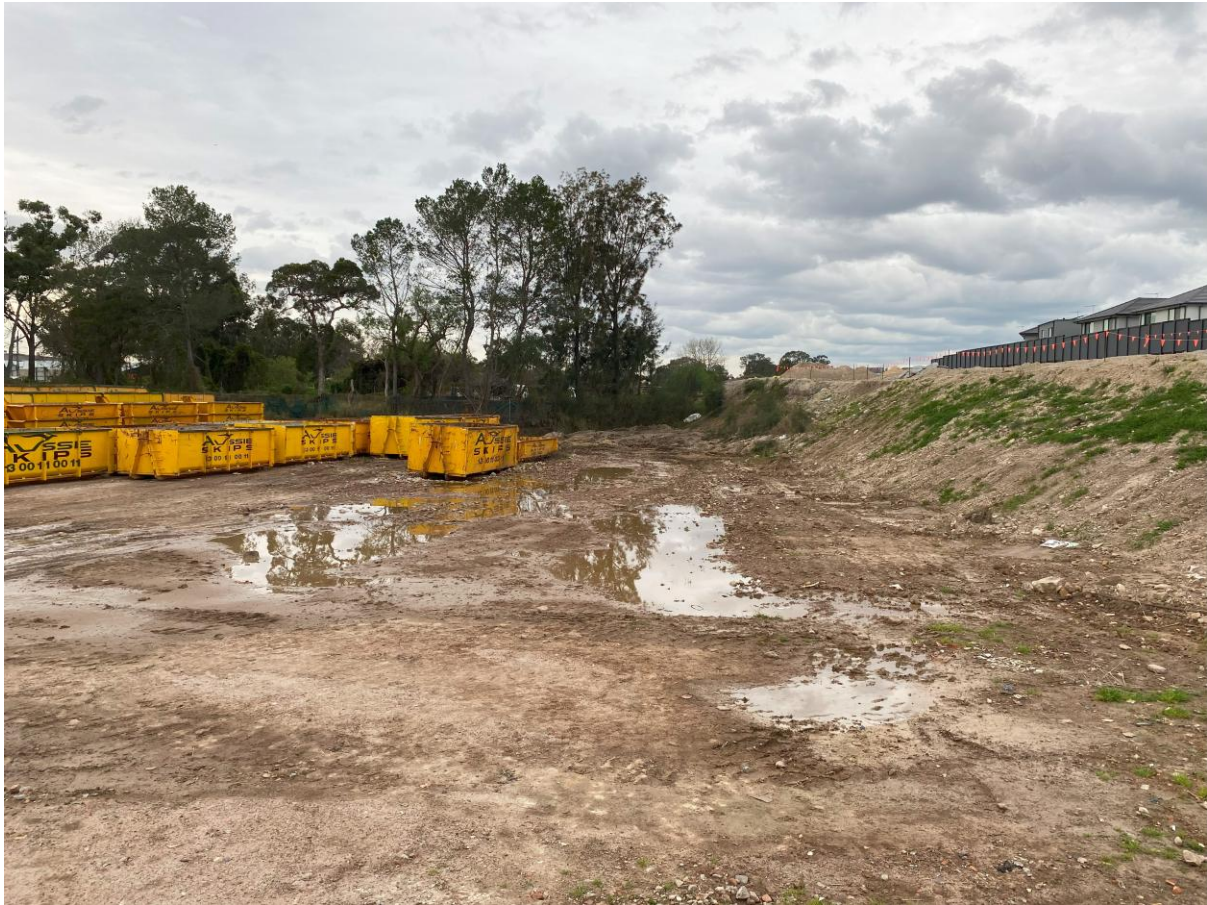
Plate P1. Ponding from recent rain on ground surface, clay soil exposed, skip bins stored to left of image.
